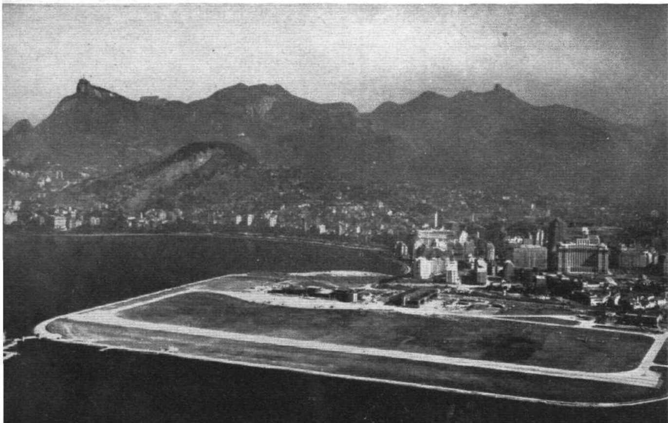
Santos Dumont Airport, Rio de Janeiro. The tall buildings in the foreground occupy the former site of a mountain levelled to supply earth for constructing the airport.
